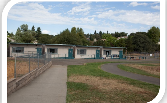
Portables need to be replaced
